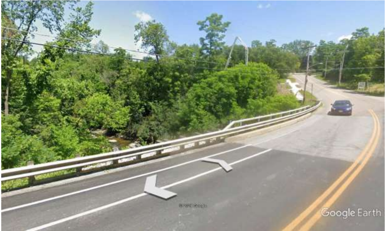
Photo from bridge facing northeast in area of pedestrian bridge. Existing sideealk can be seen in right part of photo.
