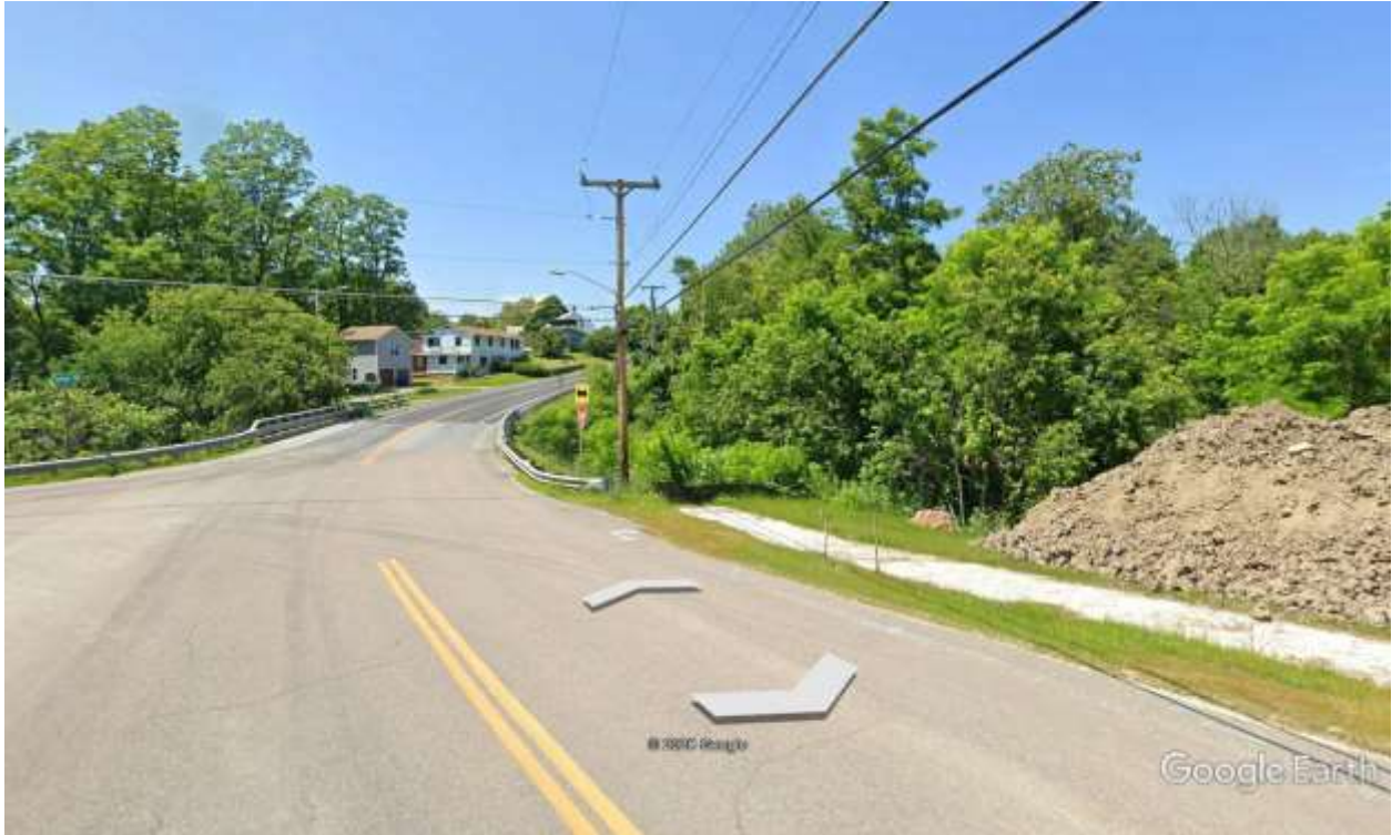
Location of proposed pedestrian bridge facing west. Existing sidewalk in foreground.
